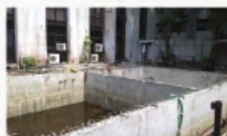
Concrete test tube tanks
