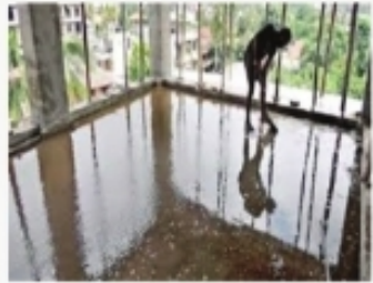
Stagnant water (concrete slab)
