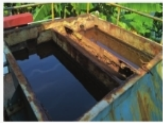
Water storage tank
